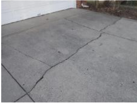
#1 Typical cracks
