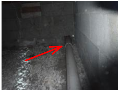
#53 Main sewer drain line
