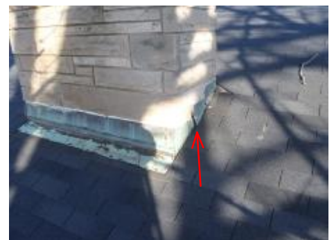
#12 Loose flashing
