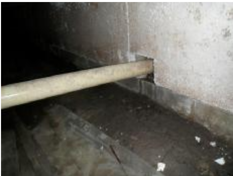
#55 Main sewer drain OK
