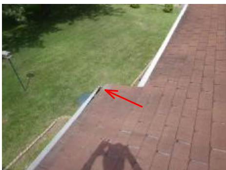
#22 Loose gutter
