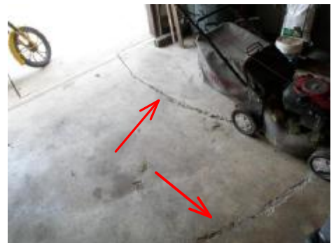
#36 Large cracks
