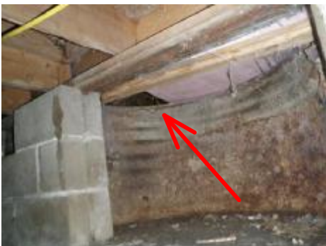
#58 Access below the deck is allowing coons ect. into the crawl space.
