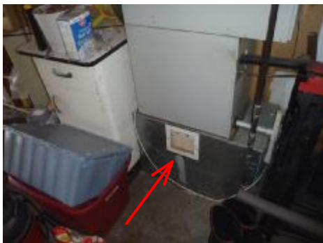
#31 Heat grill should be self closing.
