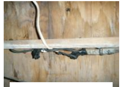
This # 12 wire in on a 125 amp breaker
