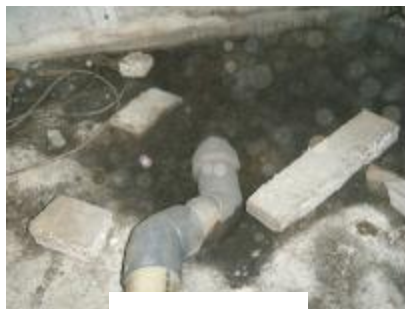
Main sewer drain line
