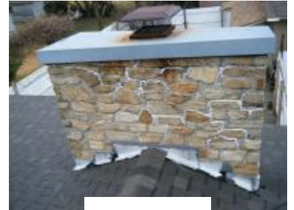
Fill cracks in mortar
