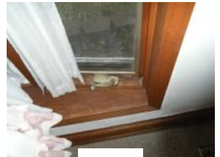
Broken crank
