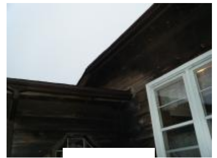
Cover soffit at peak
