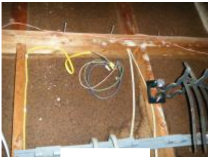
Install junction box
