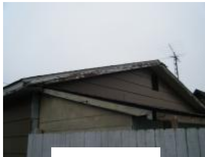
Scrape and paint wood
