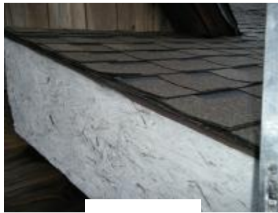
2 layers of roofing
