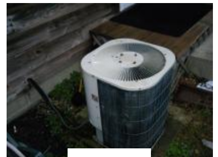
AC not inspected
