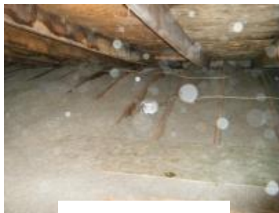
Needs additional insulation
