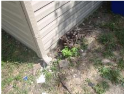
#2 Remove stump. Install splash blocks
