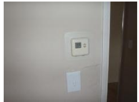
#54 Thermostat would not go lower than 77 degrees
