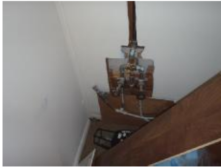
#38 Back of tub/shower inside closet
