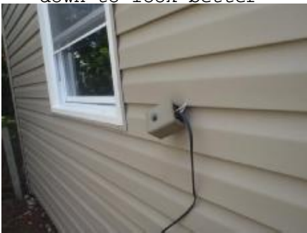
#4 Secure phone line. Phone line is on the ground
