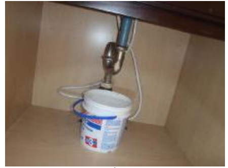
#63 Leaking trap
